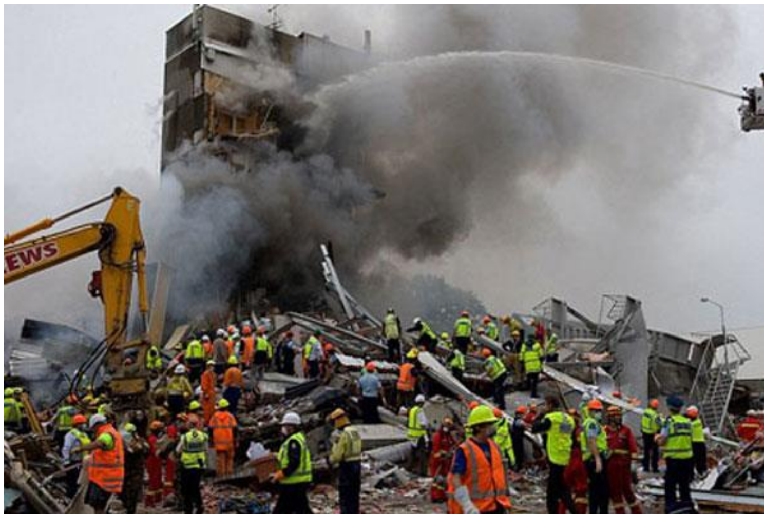
CTV building collapse
