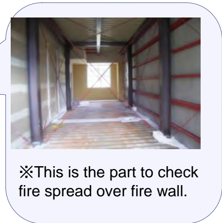
Simple steel structure
